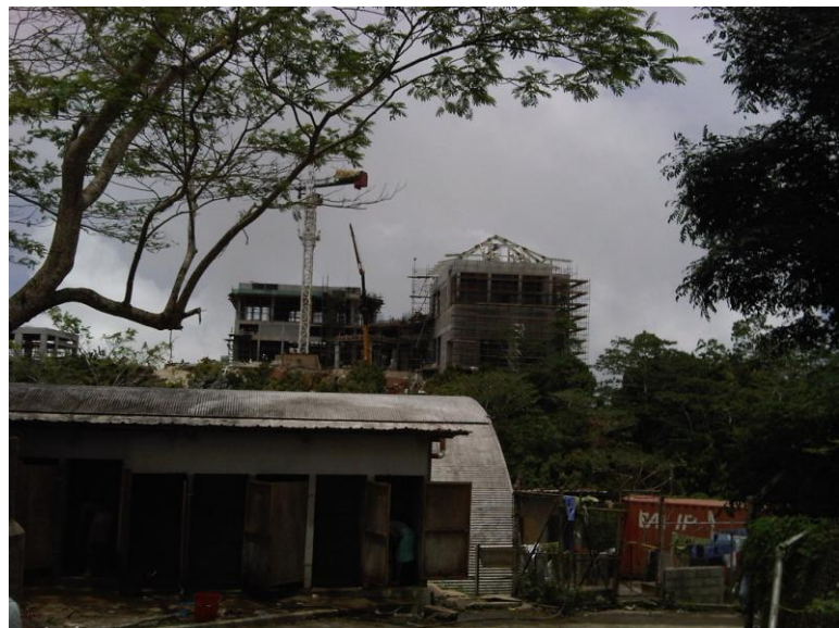
Figure 5 Construction site near La Misère.
